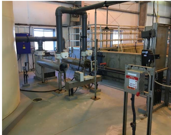
Figure 4-2. Existing UV Unit to be Removed and Replaced with a New UV System
